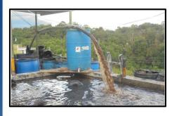
The GEM System was installed after Sedimentation Basins. To save chemical costs and achieve maximum removal rates, pH was adjusted to approximately 7.5 in a modified Equalization (EQ) Tank by adding nitric acid at 2%.
